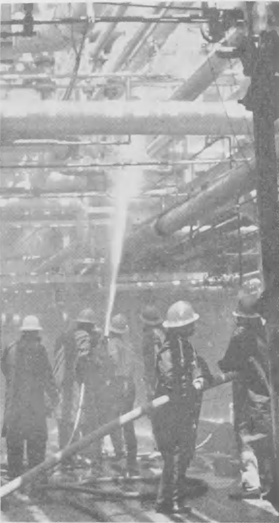
MINUTES AFTER the general alarm was sounded on May 7, the volunteer firemen were on the job at the PCAR, to cool the unit and to stand-by when the unit was being taken off stream. The unit had to be taken out of service because of a leak. Escaping products vaporized appearing as smoke.
